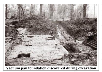
The clarified, strained syrup or molasses was then placed in a closed vessel known as a vacuum pan, where it was boiled until the sugar in the syrup was crystallized. The vacuum pan operated with steam running through copper tubing inside the pan to heat the juice. During excavation, the location of the Ashland vacuum pan was identified in Area B. A number of
