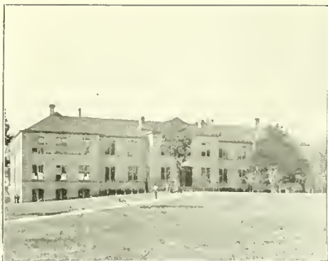
MAIN BUILDING, LOUISIANA INDUSTRIAL INSTITUTE, RUSTON, LA.
