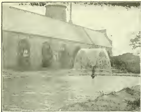
FOUNTAIN PRODUCED BY NATURAL PRESSURE FROM 3" WELL AT REISER'S MACHINE SHOP, LAKE CHARLES.
